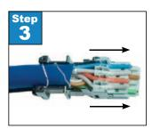
**Step 3.** Insert prepared cable into loading bar by pushing the bottom wires through the appropriate holes (ref: Wiring Diagram) and pressing down on the top row of cables to be seated into their appropriate slots. Trim the excess wires.
