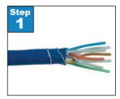
**Step 1.** After the outer sheath insulation is stripped, wrap the drain wire around the jacket. Untwist the pairs to within 1/8" of the jacket and arrange the wires according to TIA/EIA 568A or 568B standards.
