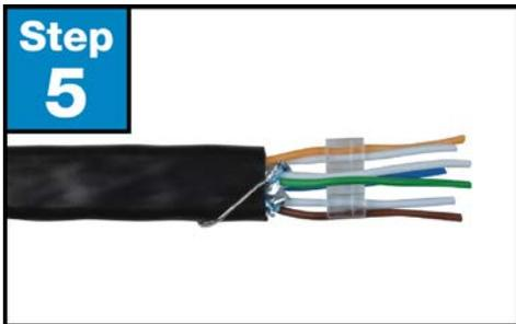
**Step 5.** Untwist the pairs to within 1/8" of the jacket. Arrange the wires according to TIA/EIA 568A or 568B standards. Slide the 1st and 4th pair of wires into each side of the cross-shaped loading bar, with the 2nd and 3rd pair respectively touching the top and bottom crevices.
