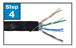
**Step 4.** Using a wire cutter, carefully clip the foil shield insulation around the each twisted pair and remove it as close to the cable jacket as possible. Do not remove any insulation from the conductors.
